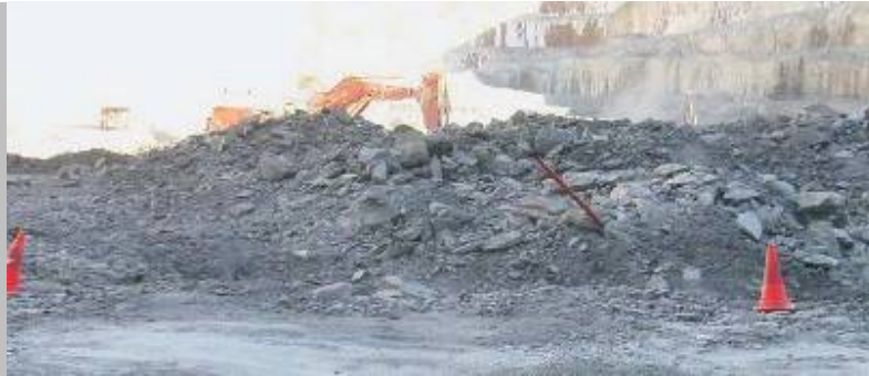
Shock tube blast muck pile.
