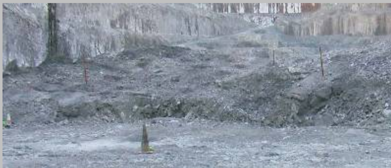
Electronic blast muck pile.
