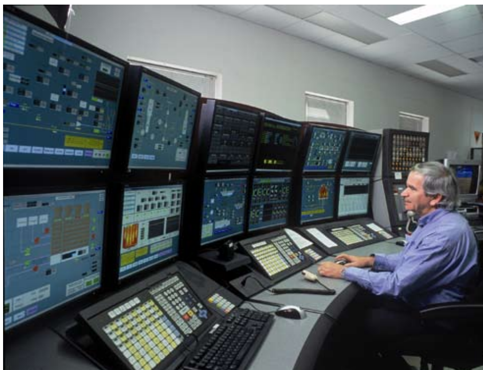
Orica uses sophisticated plant process control systems to monitor energy use at Kooragang Island
