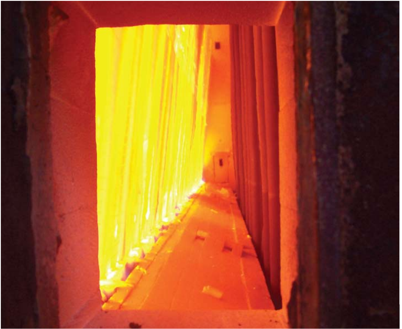
The glowing furnace refractory seen through an inspection hatch
